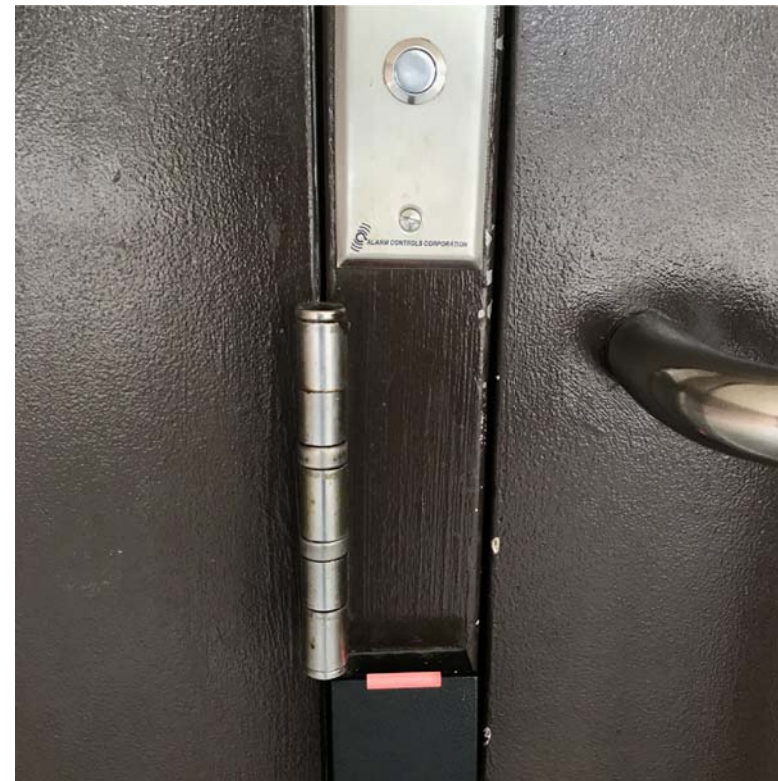
4 MAINTAIN EXISTING EXTERIOR STOREFRONT AND SECURITY CONTROLS
